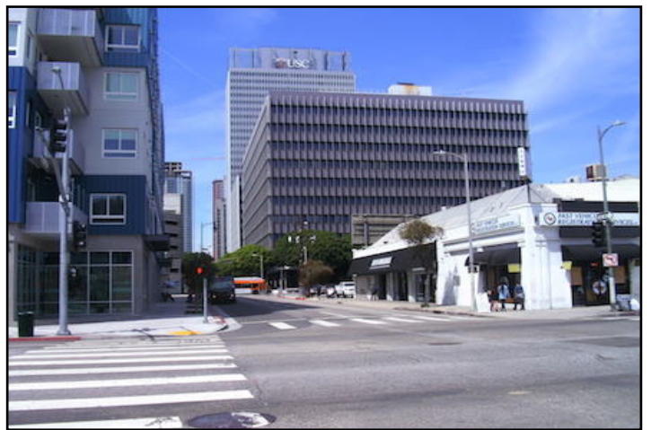
View 4: From the southeast corner of the intersection of Main Street and 12th Street, looking northwest at the southern border of the Project Site.
