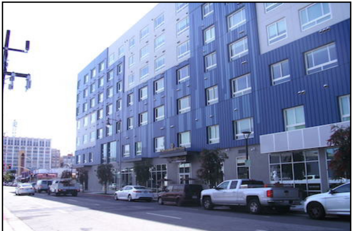
View 12: From the north side of 12th Street, looking south at the commercial buildings adjacent to the Project Site.
