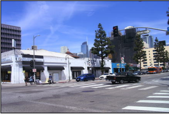
View 1: From the southeast corner of the intersection of Main Street and 12th Street, looking north at the Project Site.
